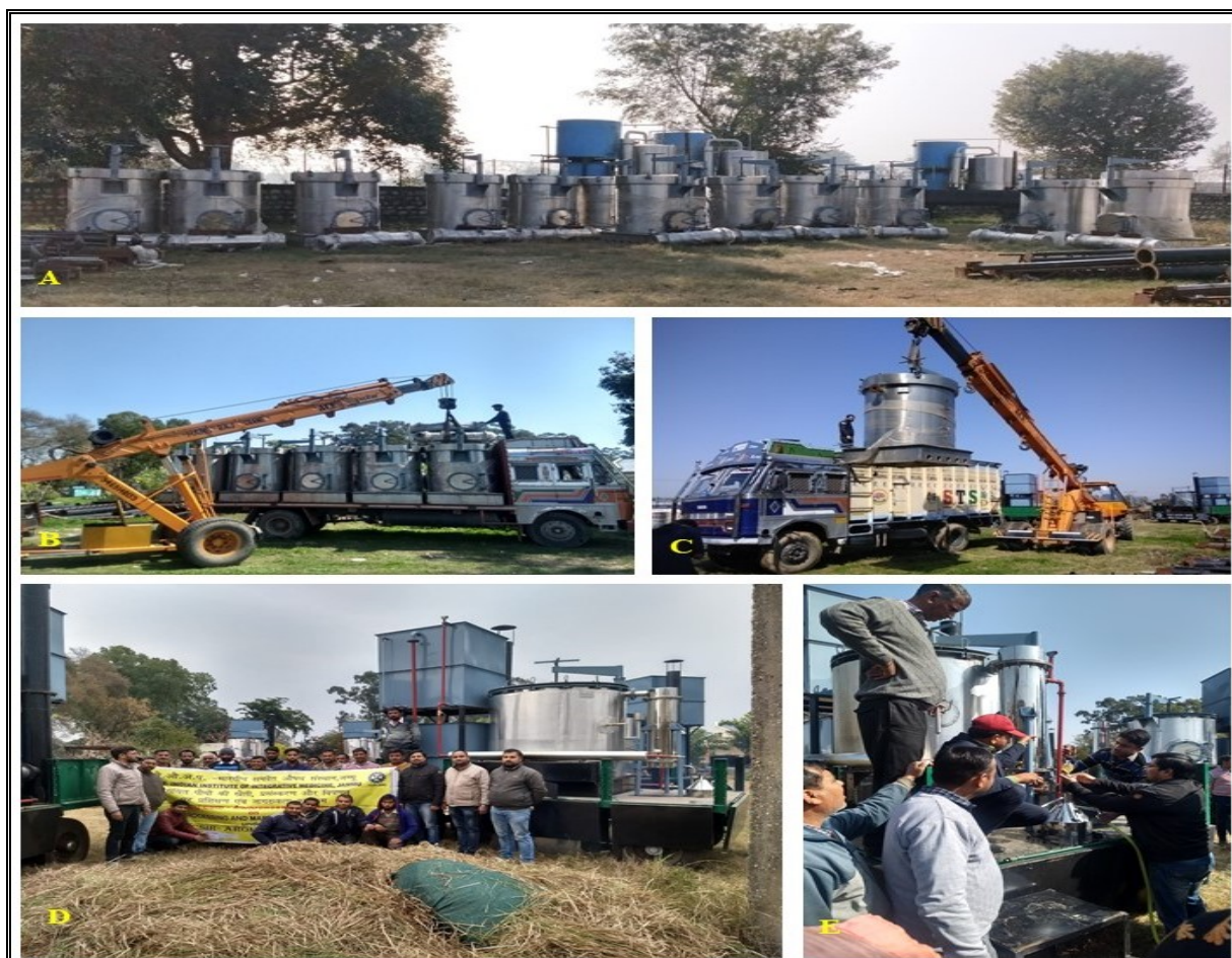
Figure SA1.2. Transportation and installation of fixed and mobile Distillation Units under CSIR-Aroma Mission.
